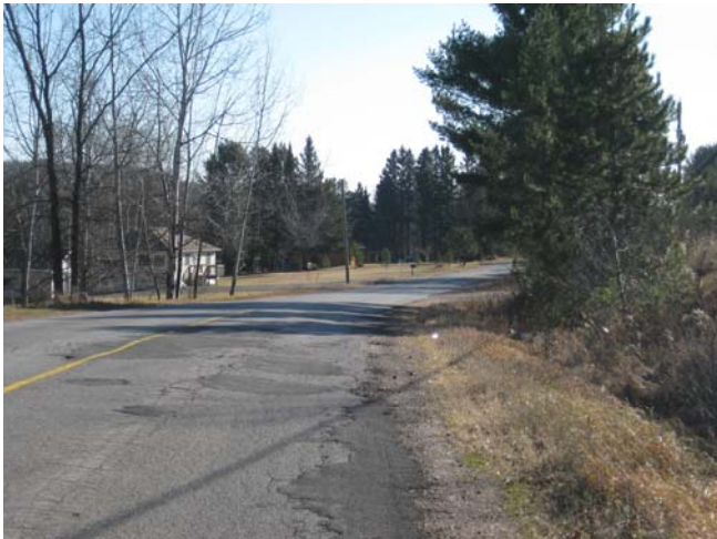
Typical conditions illustrating poor pavement condition, lack of shoulders, roadside hazards/visibility (i.e. trees)
