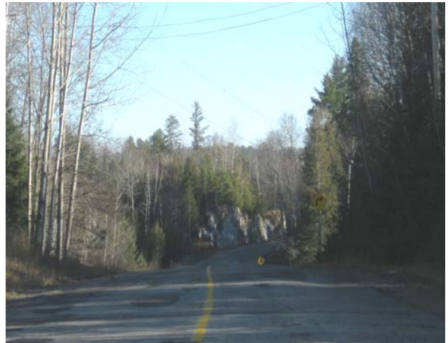
Photo illustrating sharp horizontal and vertical curves, reduced visibility, and adjacent rock outcrop
