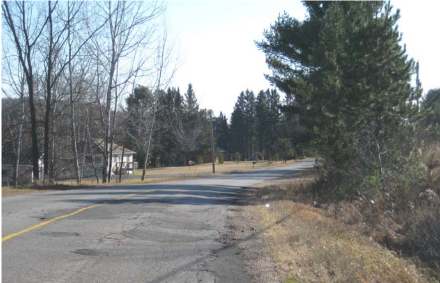
Typical conditions illustrating poor pavement condition, lack of shoulders, roadside hazards/visibility (i.e. trees)
