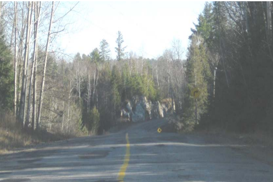
Typical conditions illustrating poor pavement condition, lack of shoulders, roadside hazards/visibility (i.e. trees)
